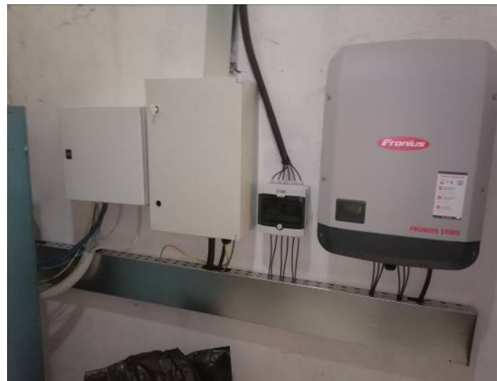
Page 8 and 9 Electric vehicle charger and PV installation Inverter
